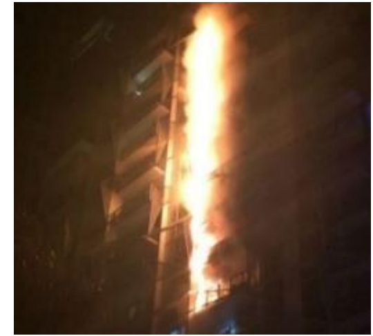
Lacrosse tower fire, Melbourne
